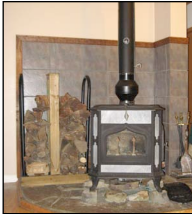
The original DRAW COLLAR on a wood burning stove with vertical output.
