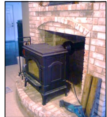
The original DRAW COLLAR on a wood burning stove with horizontal output.
