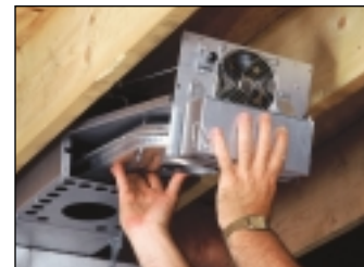
Install Venter Assembly
